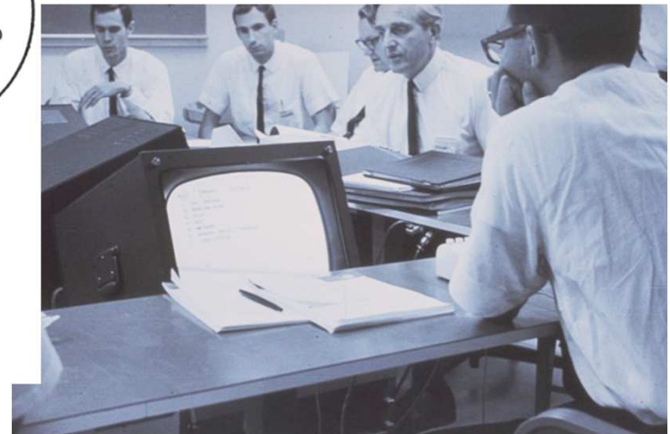
Network terminal (end of sixties)
