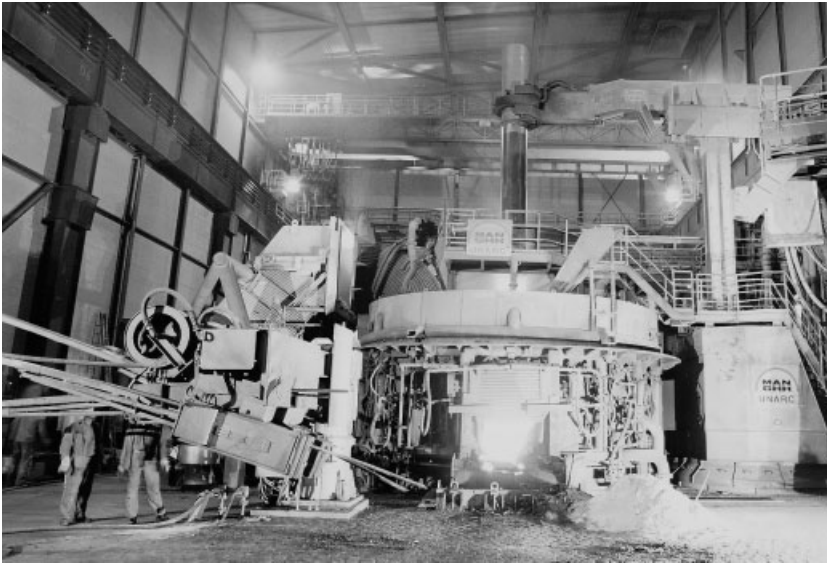
Figure 17. 100-t-steel melting direct-current arc furnaces, type UNARC (courtesy of MAN GHH).
